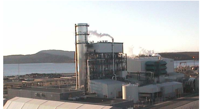
Fig. 5: The NGCC Power Plant at Kårstø, West Norway.
