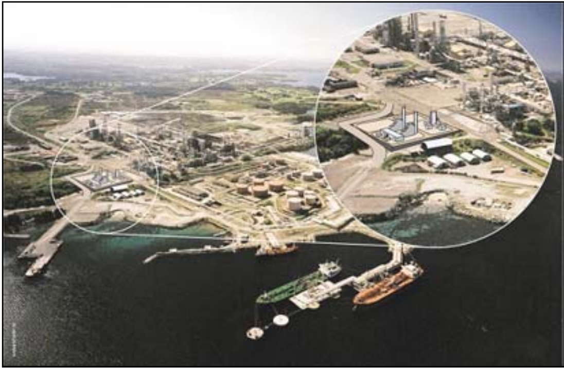
Fig. 9: Mongstad refinery is at present the single largest emission site for CO 2 in Norway. In 2006 it will emit ~1.7 mtCO 2 /yr. Also, Mongstad Energiverk is proposing a 240 MWe (320 MWth) combined heat and power (CHP) plant (see insert) so that total CO 2 emitted from the refinery and the CHP plant may then be 2.3 mtCO 2 /yr.
