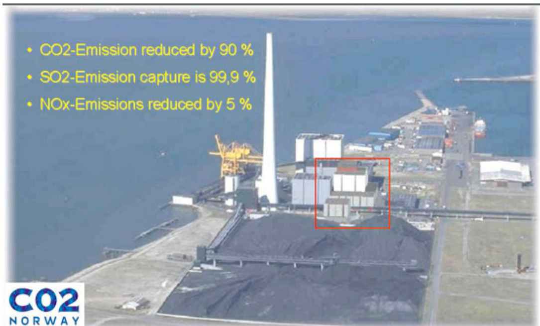
Fig. 5: Aerial view of the Elsam coal-fired power plant Esbjergværket including an artist impression of the CO 2 -capture plant (within the red square). The smaller building (nearest, on this side of the road) houses the CO 2 compressors, while the large (mostly white) building is the amine plant. The grey building immediately adjacent to the left, is the existing plant for Flue Gas Desulphurisation (FGD).
