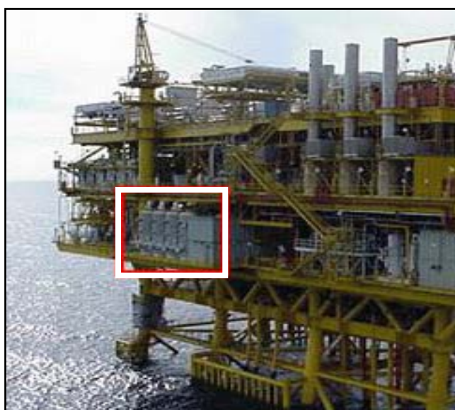
Figure 5: A CO 2 -membrane stripping unit (high-lighted) attached to an offshore platform operated by Unocal in the Gulf of Thailand. The unit shown here is handling 1,8 mtCO 2 /yr.
