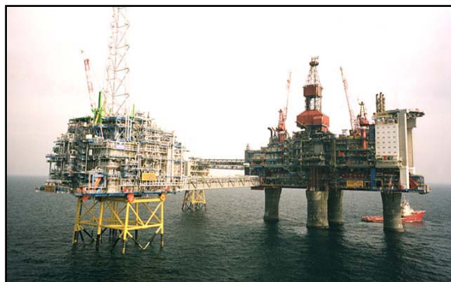
Fig. 4: The Sleipner-T (CO 2 amine-treatment) and Sleipner-A (production) platforms, where one mtCO 2 /yr are currently treated and injected by Statoil as part of a pilot study on saline aquifer storage in the North Sea.
